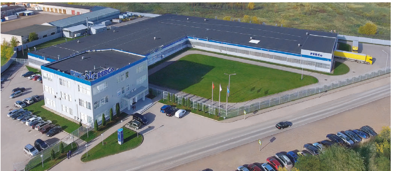
PERCo manufacturing plant
